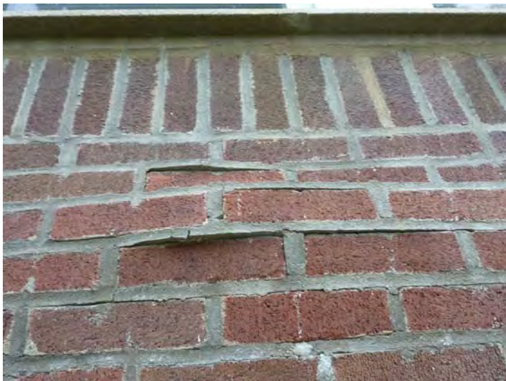
Eccentric brick failure is shown to be repaired in Year 1.
