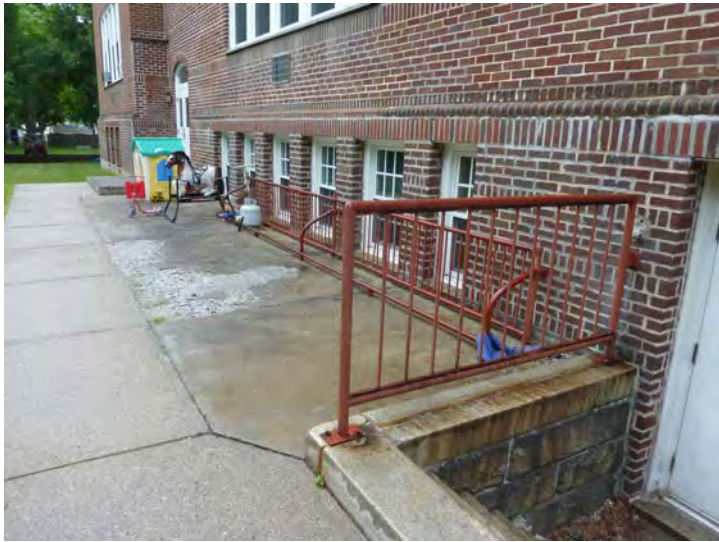
Failing concrete pad is shown to be replaced and rusting steel handrail and bike rack is shown to be painted.
