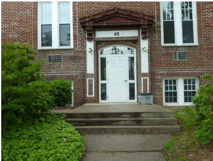
Trip hazards at concrete pavement leading to front door and at all other locations site wide are to be eliminated in Year 1.
