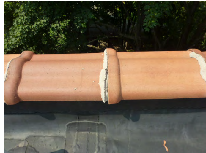
Failing joints and finish of clay tile coping at select locations are shown to be repaired in Year 1.
