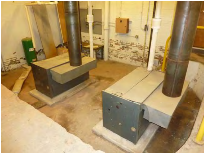
Signs of historic water damage at the brick basement foundation walls at the building hot water boiler pit. Boilers are shown to be replaced in Year 1.
