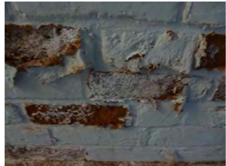
Typical historic water damage at the brick basement foundation walls is shown to be repaired in Year 1 and periodically during the plan.
